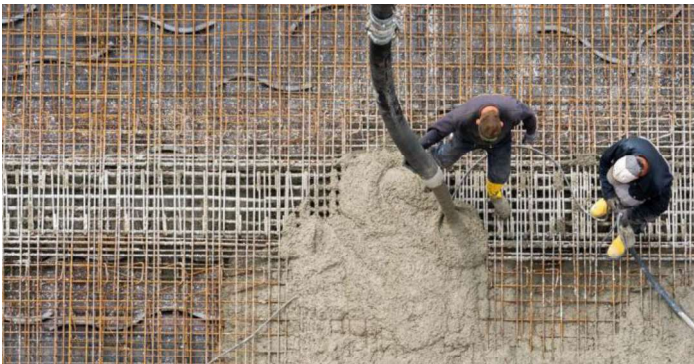
Figure 1: Use of Steel Reinforcement on the Construction Site for Concrete Pouring
